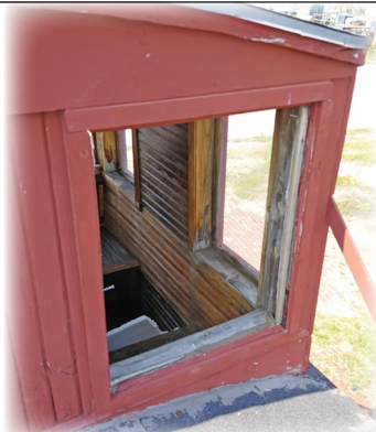
Above: Window in the cupola of the caboose that was broken by vandals, who also scattered trash in the train car.
